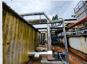
Cooling/Chill water pump
